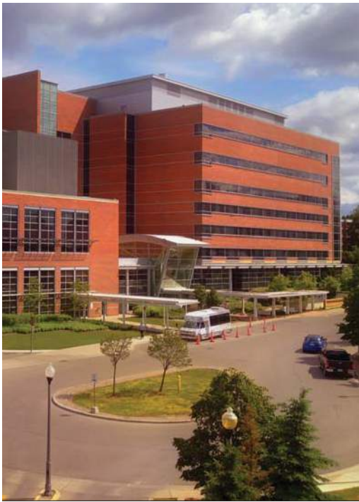
(Above) Lakeridge Health hired Ecosystem to increase energy efficiency, renew assets and improve the patient experience at all four of its Ontario hospitals through 29 different measures fully funded by incentives and energy savings.
