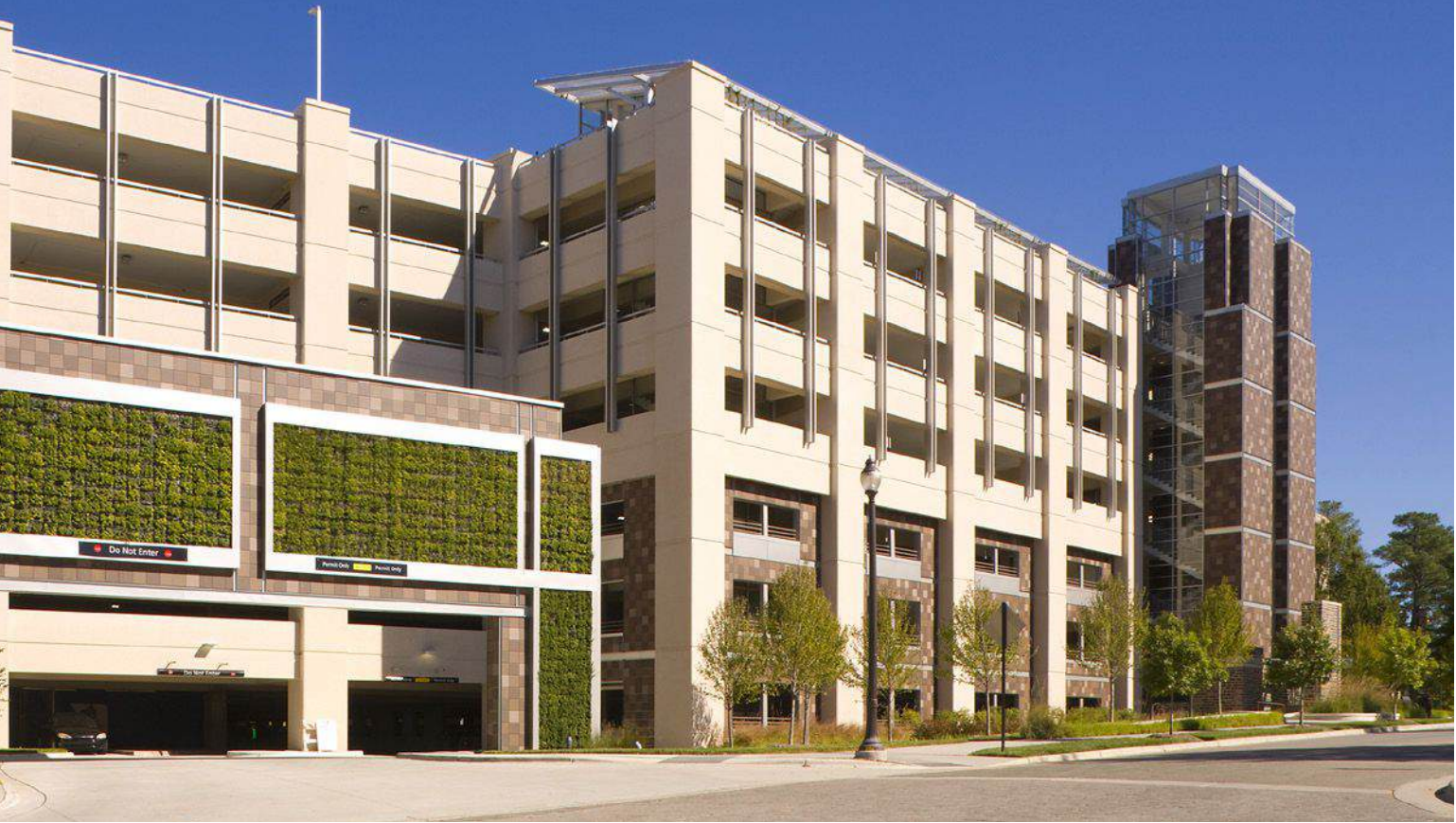
An exterior express ramp on one side of Duke University's Research Drive Parking Garage allowed all the floor plates to be flat, providing passive security with unobstructed internal views. Photo: Ratio.
