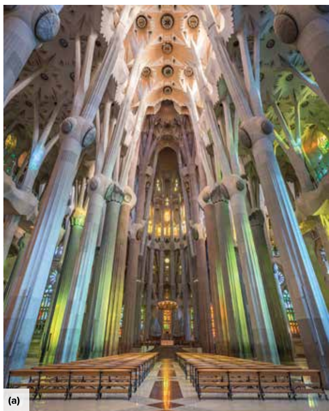
Fig. 4: The interior of the cathedral is a celebration of light: (a) Tree-like columns and their “branches” line the main nave, seen here looking toward the apse. Four types of columns have been constructed: columns on each of the four corners of the crossing support the Jesus Christ tower and partially the weight of four Evangelist towers; columns that bear the main load of the four Evangelist towers; columns in the apse and naves; and columns that separate the side naves from the main nave; and (b) The longitudinal nave on the Nativity façade side of Sagrada Família features stained glass windows that gradually transition from yellow to green to deep blue (© Fundació Junta Constructora del Temple de la Sagrada Família)
