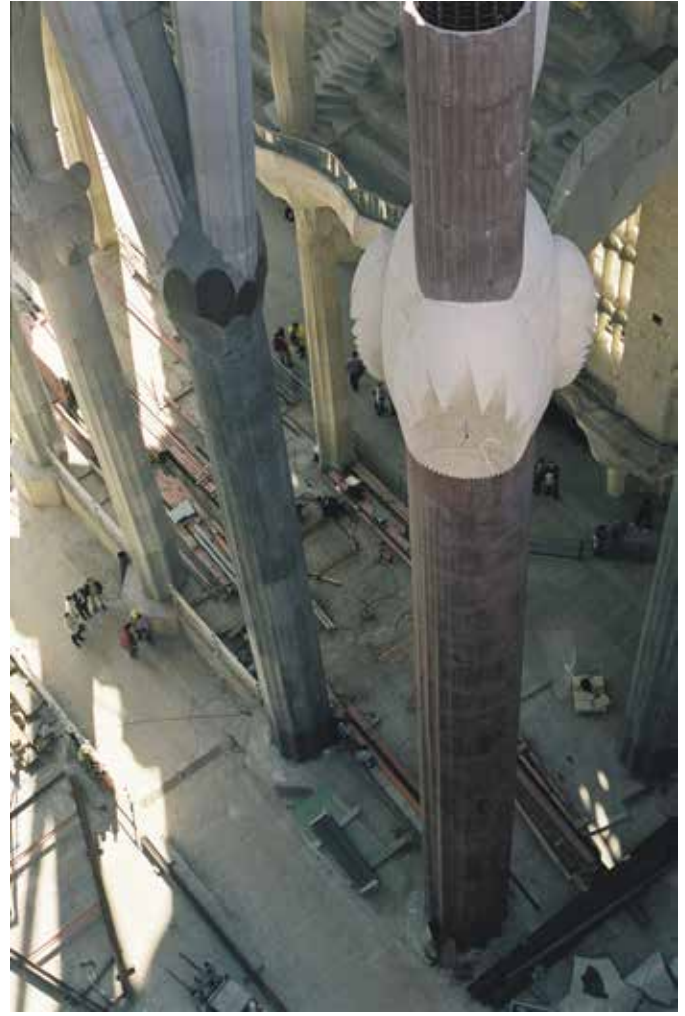
Fig. 6: Stone or precast concrete exterior “drums” were used to form the trunks and branches with reinforced concrete cores (© Fundació Junta Constructora del Temple de la Sagrada Família )
