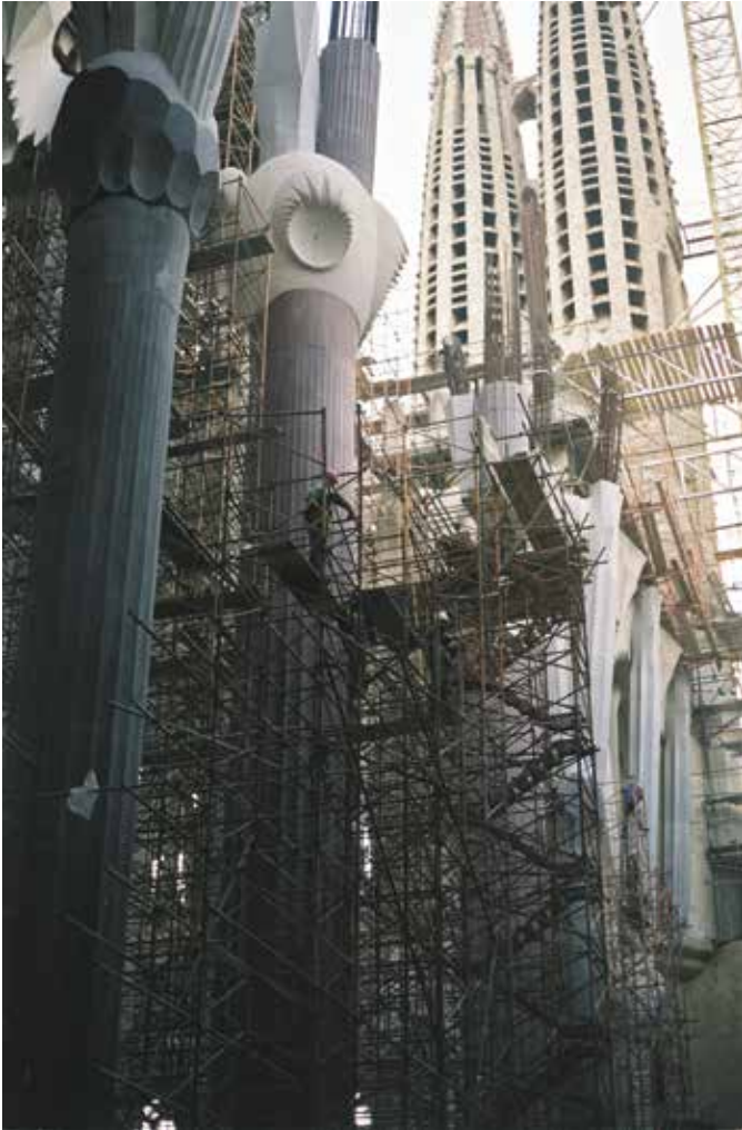
Fig. 6: Stone or precast concrete exterior “drums” were used to form the trunks and branches with reinforced concrete cores (© Fundació Junta Constructora del Temple de la Sagrada Família )
