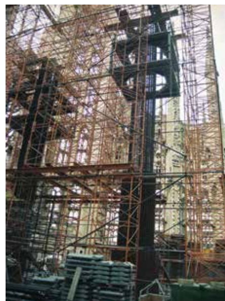
Fig. 5: Construction of the interior columns was completed inside the existing façades between 1991 and 2003 (© Fundació Junta Constructora del Temple de la Sagrada Família)
