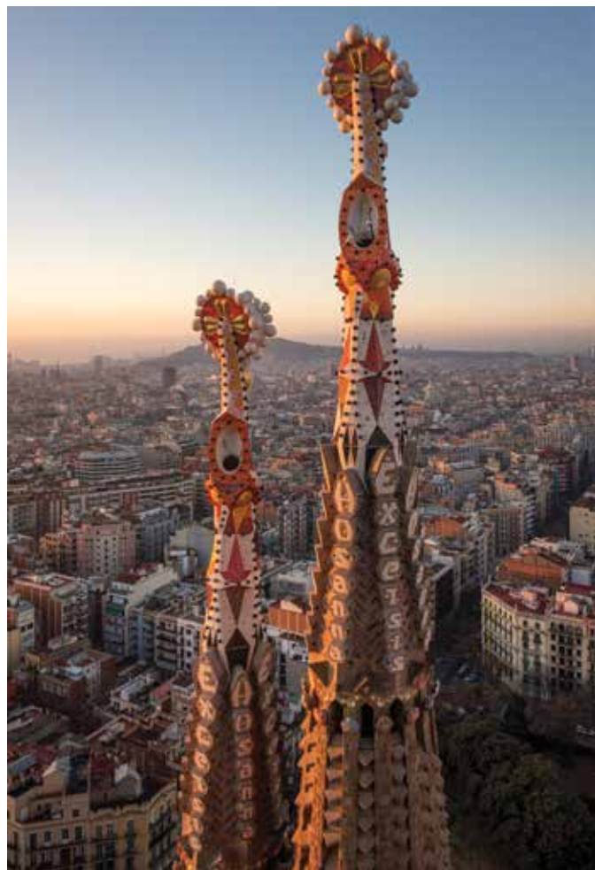
Fig. 3: Close-up of two pinnacles of the Passion façade spires. The towers are decorated with mosaic tiles (© Fundació Junta Constructora del Temple de la Sagrada Família)
