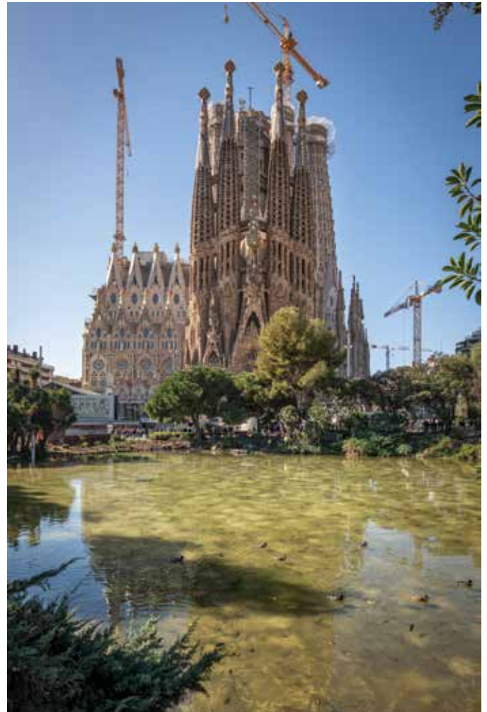
Fig. 1: The Nativity façade features two 107 m (351 ft) towers flanked by 98 m (321 ft) towers. This façade was nearly completed under the direction of Gaudí (© Fundació Junta Constructora del Temple de la Sagrada Família)
