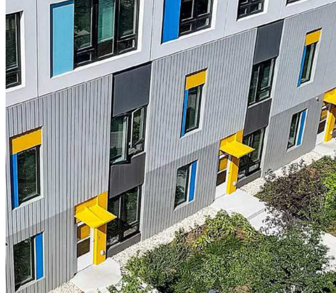
The first two floors of the Lucy Gonzales Parsons Apartments complex feature texturing that mimics shiplap siding. Wells used formliners to achieve the textured panels. Recessed colored panels around the windows were designed to look like part of the window frames. Photo: Wells.
