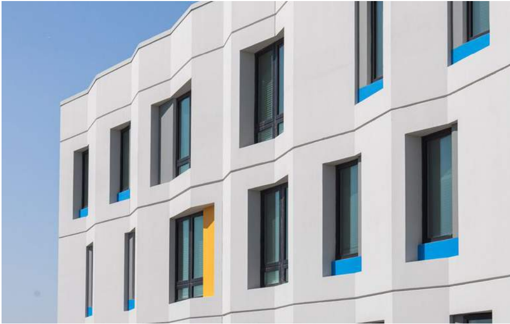
The middle section of the apartment complex features precast concrete panels that are flat on the interior but bump out about 2 ft on the outside to provide an architectural ripple in the building's exterior. Photo: LBBA.
