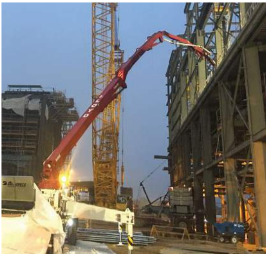
"The concrete pump knows if the mix doesn't have enough water," says Steve Lloyd, "and it won't pump without water." PHOTO: LLOYD CONCRETE SERVICES
