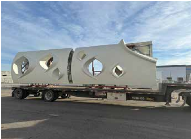
Fig. 5: Finished GFRP panels were transported on a truck from Salt Lake City, UT, to Denver, CO (photo courtesy of Cannon Masonry)
